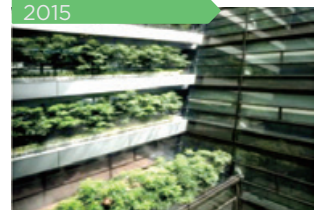
④ The SHASE Awards Dry mist facilities (The company that designed the building won the award for its air-conditioning technologies)
