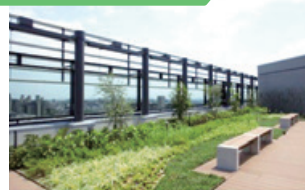
③ Rooftop and Wall Greening Technology Contest Greening the rooftop
