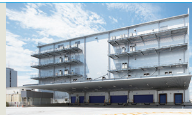
The view of the No. 2 Logistics Building
